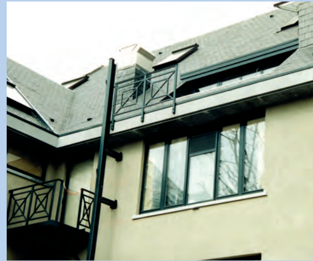
Guardrail with custom design
