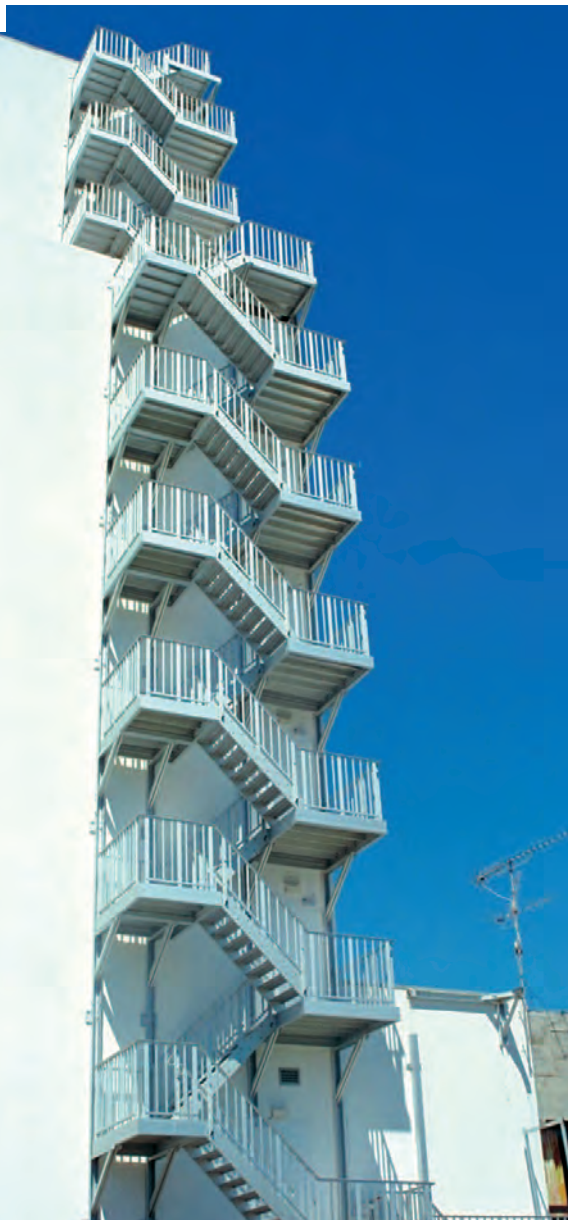
Stair suspended from the façade
